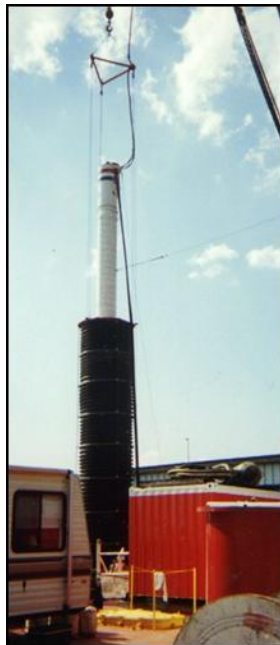
Figur 6: Avskärmning av pålning, exempel 3 (U.S. Department of Transportation - Research and Innovative Technology Administration, 2006)
